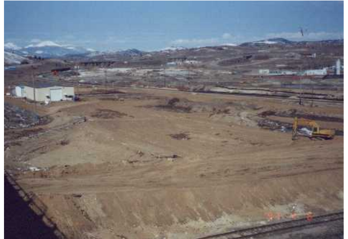
North side backfilled with clean overburden
