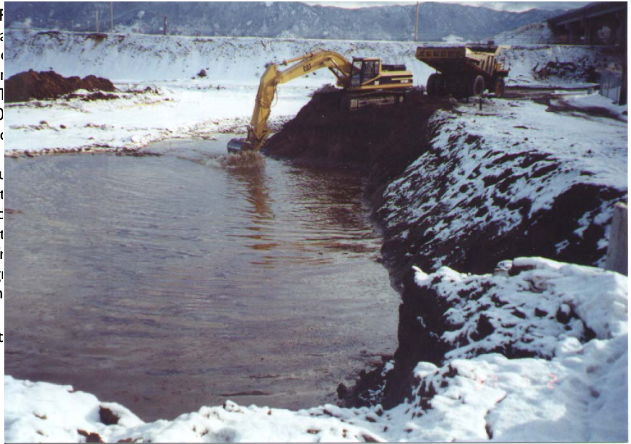
North side excavation
