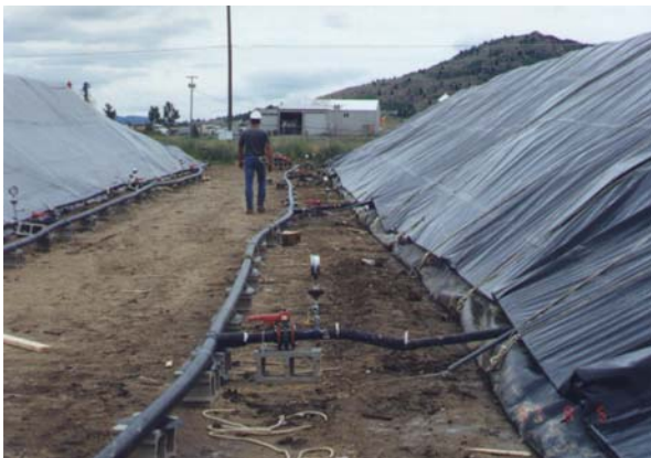
Soil staging and pre-treatment piles
