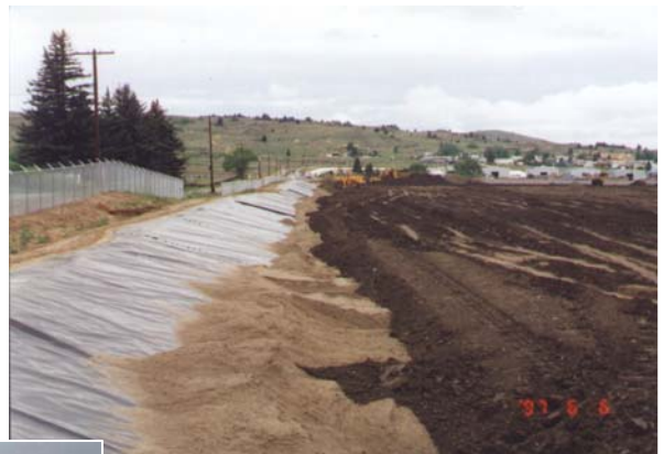
Excavated soils placed on the land treatment unit for biological treatment of contaminants
