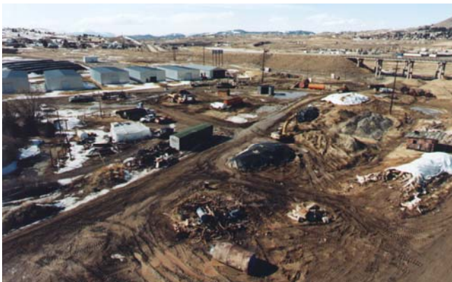
Site debris before remediation
