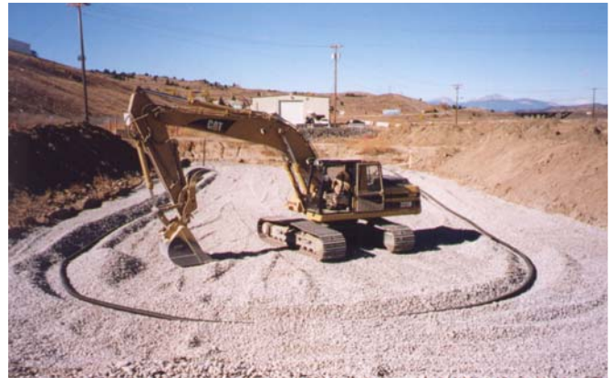
North side piping and gravel in situ treatment system, Phase 3
