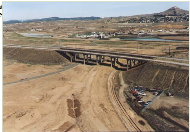
Bridge work will provide clean cover soil for Montana Pole
